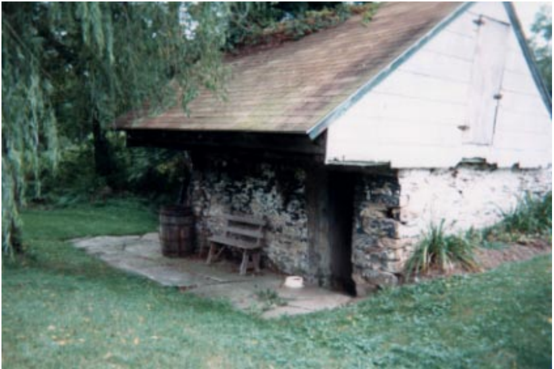
This is the springhouse on the farm of Hans and Anna Wenger. It was the first structure built upon settling on the land. The old wooden roof shingles were replaced with modern day asphalt shingles a number of years ago. A strong flow of water still takes place in the old spring house.
